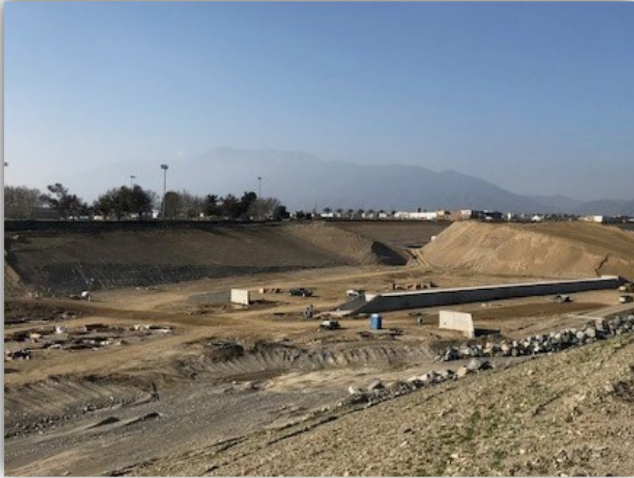
Figure 4 Photograph of Upper Cactus Basins Rehabilitation Project
