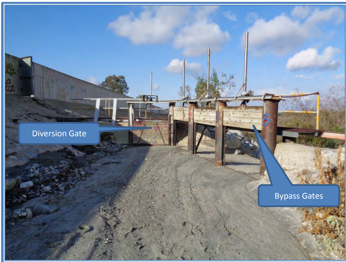
Figure 6: Mill Creek Diversion Headworks (Looking West)
