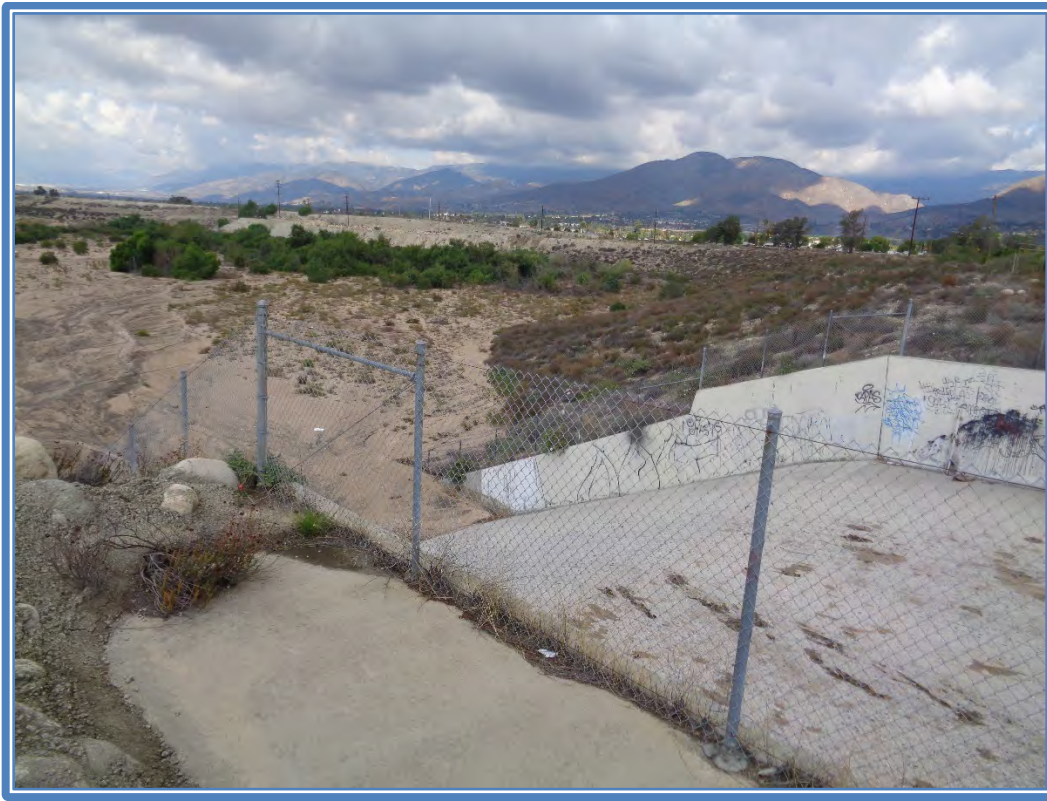
Figure 17: Plunge Creek Basin 1 Site (Looking North-West)
