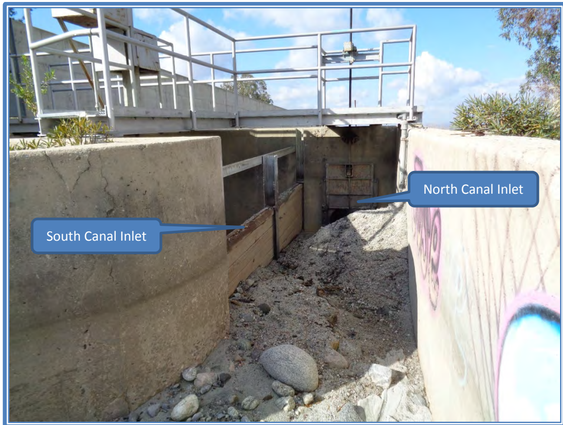
Figure 7: Mill Creek Canal Inlets (Looking West)
