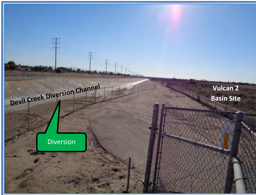
Figure 117: Vulcan 2 Diversion Site (Looking South West)
