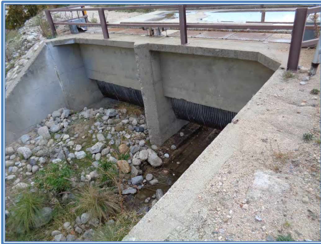
Figure 47: Waterman Basins Site (Existing Diversion Radial Gates)
