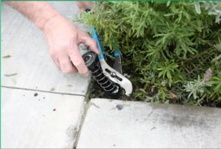
Remove the sprayhead
