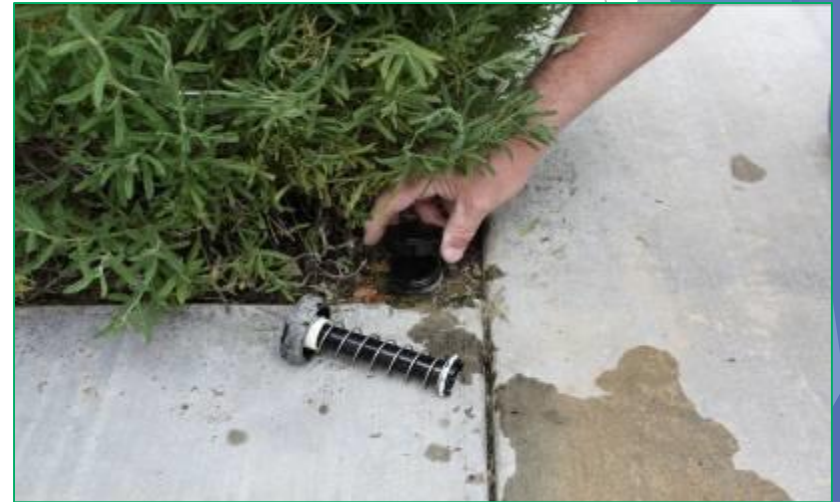
Cap off the remaining sprayheads
