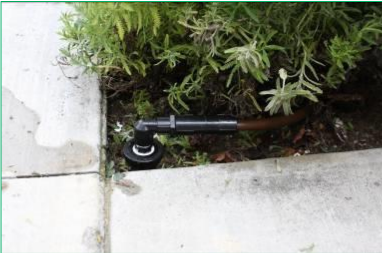
Attach the fitting & tubing
