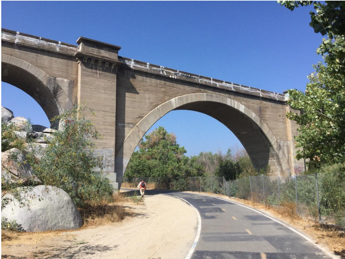
Figure 12. Union Pacific Railroad Bridge (CA-RIV-3361/H) View Toward Northwest
