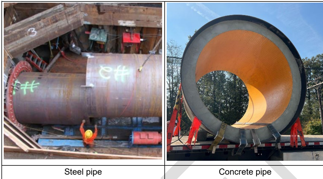
Figure 124 Suitable Jacking Pipes for Microtunneling
