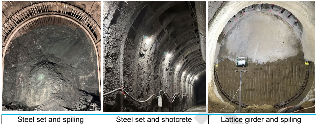
Figure 8 Example of Support System in SEM Tunneling
