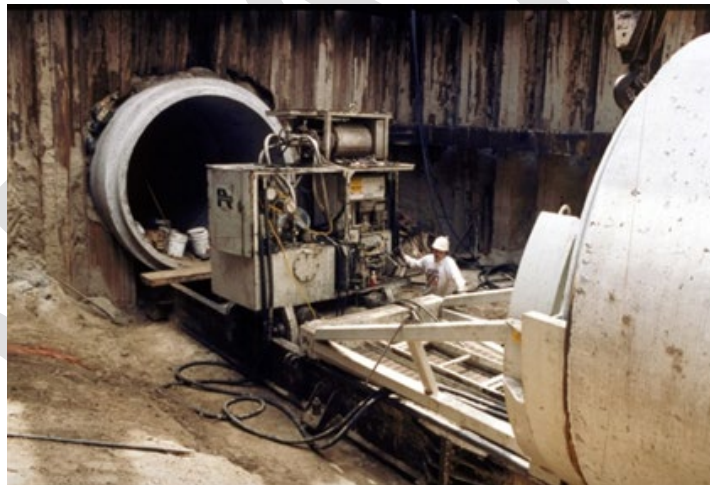
Figure 102 Pipe Jacking Shaft Set-Up
