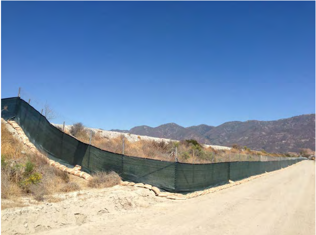
Figure 1. Photograph of Chain Link and Shade Cloth Fence Configuration
