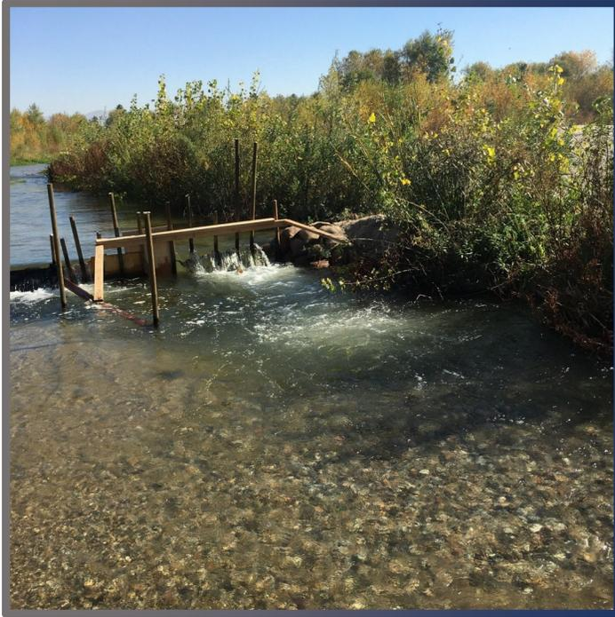
Figure 2. In-stream pilot project indicating coarse sediment downstream of flow diversion.
