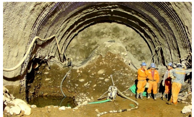
Figure 8. Boulders encountered in excavation phase.
