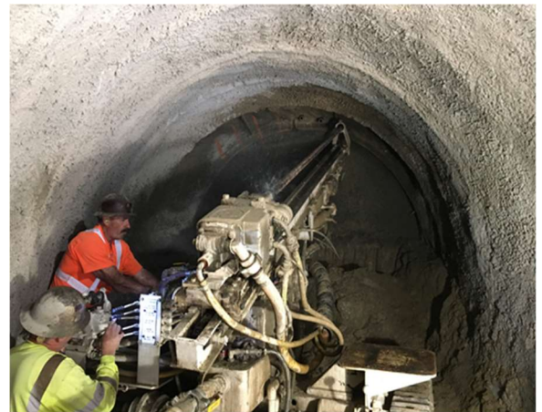
SEM Toolbox item (installation of pipe spiling).
