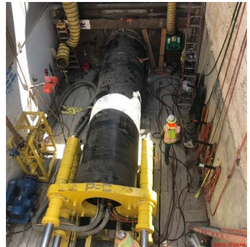
Microtunnel installation of 63-inch-diameter casing.
