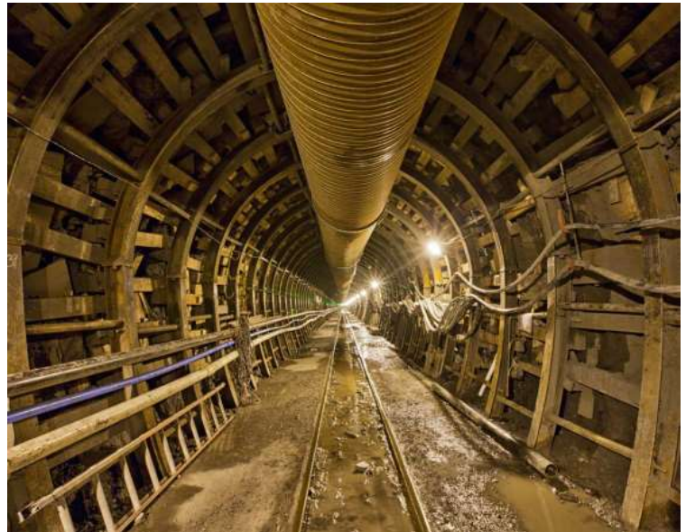
Horseshoe tunnel with rib and lag support of excavation (SOE).
