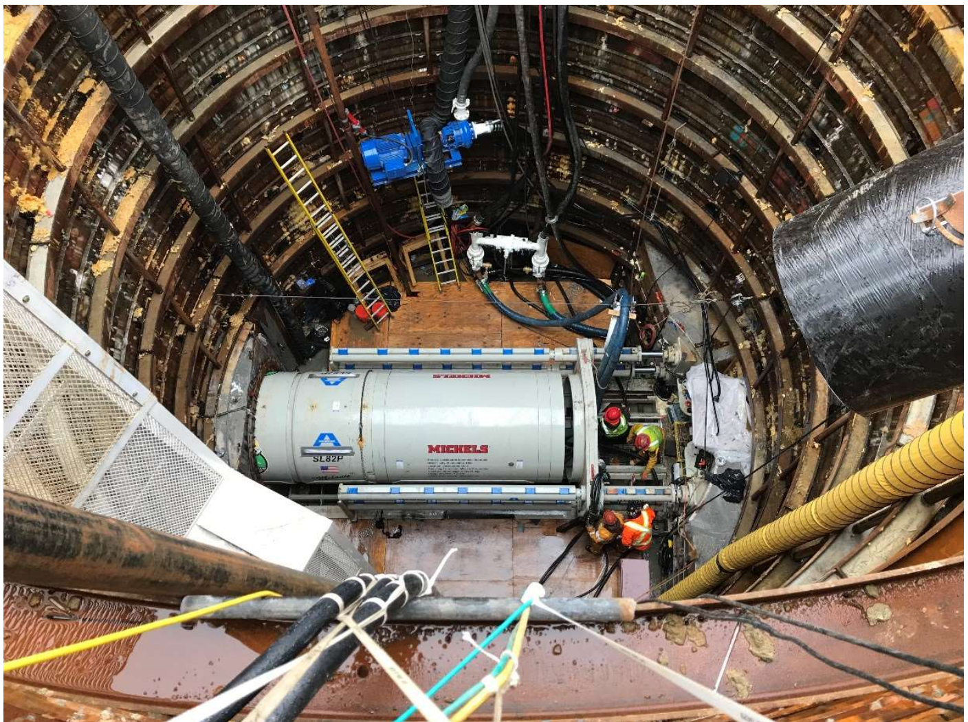
Launching of MTBM for a microtunneling drive.
