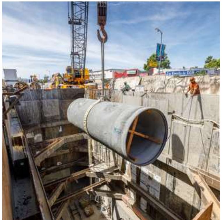
Pipe section being lowered into place at RSC Units 5 & 6.
