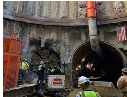
MTBM break-through into EPB Launching shaft with EPB Tail Tunnel.
