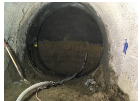
Figure 7. LADWP City Trunk Line SEM Tunnel; shotcrete application.
